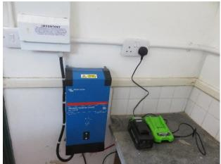
The rest of the solar system (batteries, controller and inverter), which we installed and connected ourselves, is inside the building. Lights, power sockets and a consumer unit were installed by an electrician friend who also did the final connection between the two elements. We have purchased an electric urn which had its first use when we hosted a touring side for a Sunday afternoon game in mid-August.
